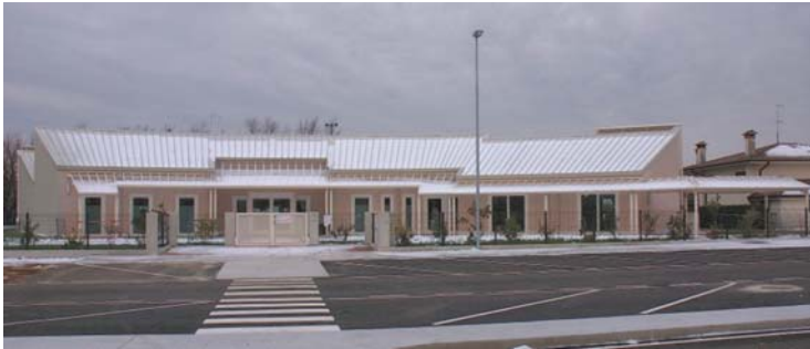
Photo n. 9 In winter, a porch on the north side, protects the wall against the effects of the prevailing winds, heavy rain and snow.
