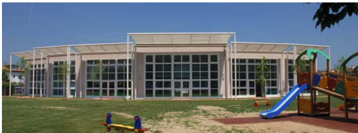
Photo n. 8 In summer the South glasses is shielded from external fixed sunscreen.
