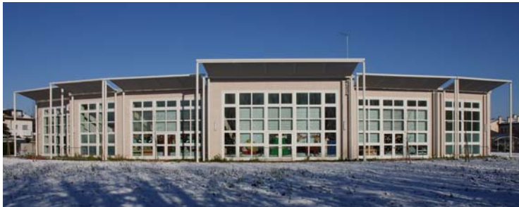
Photo n. 7 In winter the South glasses are illuminated by the Sun and the direct light is controlled by adjustable internal 'venetians'.
