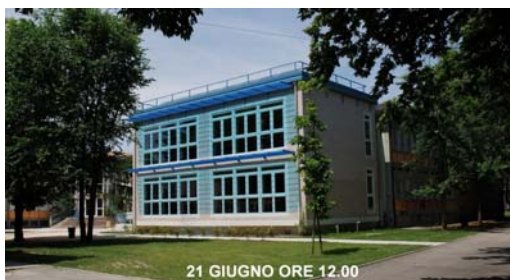
Photo n. 6 In summer the South glasses are shaded by sunscreens.
