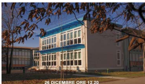
Photo n. 5 In winter the South glasses are illuminated by the Sun and the direct light is controlled by internal adjustable 'venetians'.
