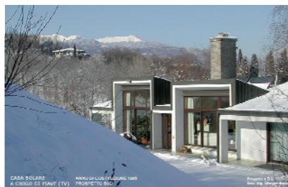
Photo n. 3-4 The building has taken very little maintenance and meets the favour of the occupants since 1985.
