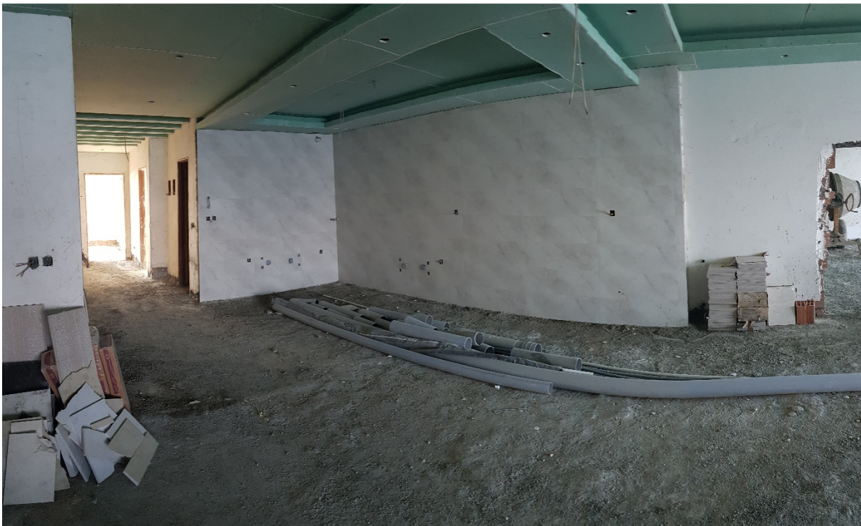
Figure 2: This is a complete view of the kitchen.
