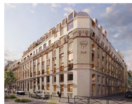
Crèche + 210 logements/210 apartments - livraison/delivery 2018 - Paris (75016) - Nexity - Carac
