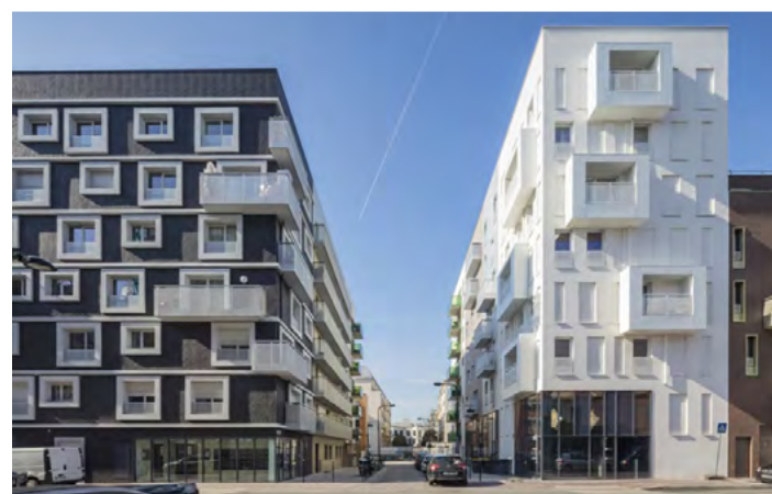
Théâtre/theater + 63 logements/63 apartments - livré/delivered 2016 - Clichy-la-Garenne (92) - LNC
