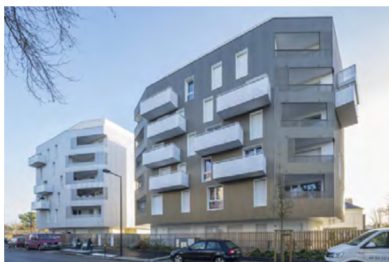
67 logements/67 apartments - livré/delivered 2016 - Rennes (35) - Giboire
