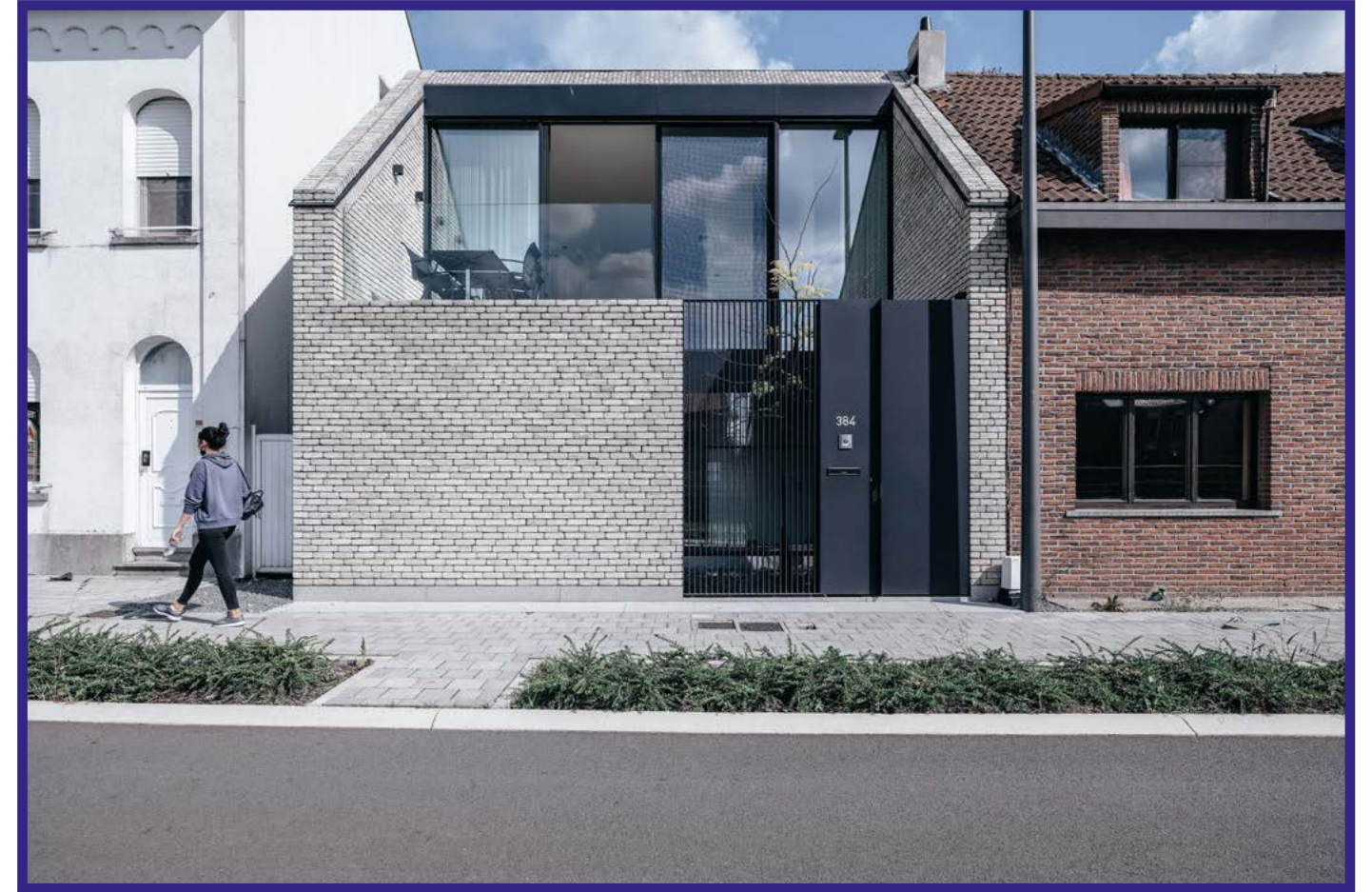
File name: PH E 010 Caption: Studio Farris Architects, Canal House Humbeek. Photo: © Martino Pietropoli.
