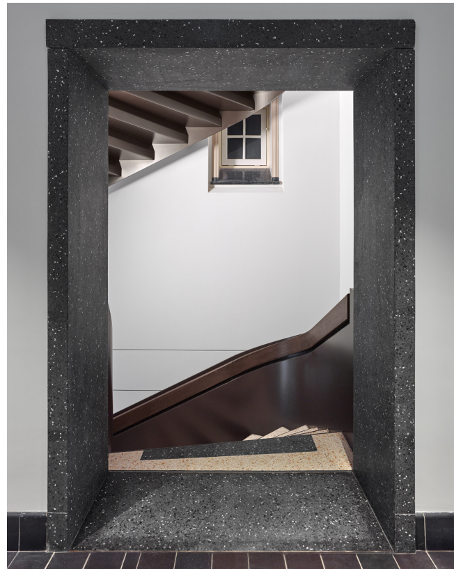
Terrazzo frames at the stairwell
