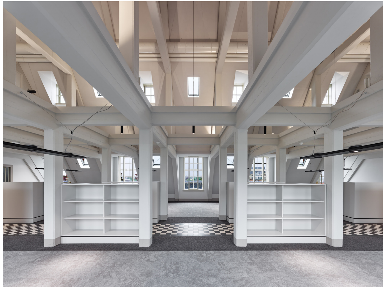
Attic with the concrete hull in sight
