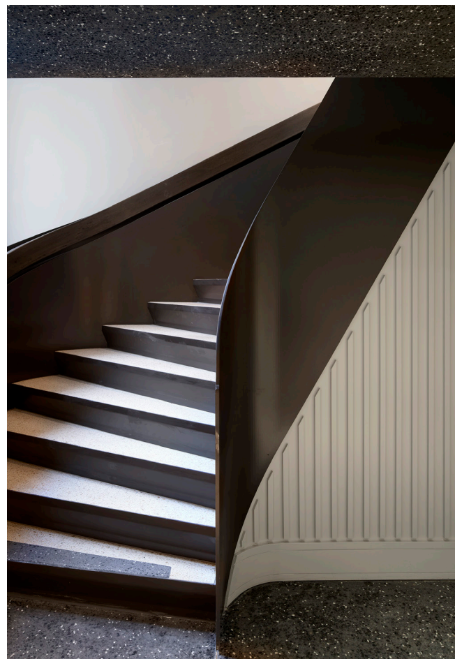
New steel staircase with terrazzo steps
