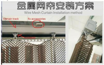
No matter the straight track or curved track, the installation method is the same(the above is the straight curtain track, below is the curved curtain track).
