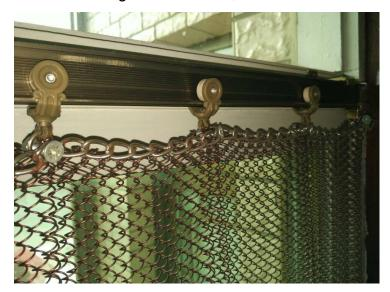
First step: you install the **curtain track** on the ceiling(or wall) with the fix accessories,these fix accessories is inside of packing,you can find there are lot of small pcs(**fix accessories**) that can hook on the track and also there is a holes can put the nail throught. Then put a nail throught the holes and fix that track on the ceiling(or wall).
