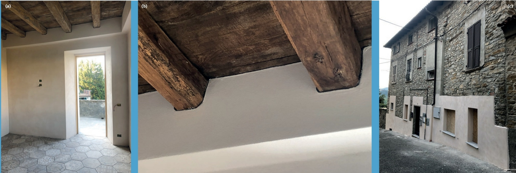
Fig. 8: (a-b) Internal insulation finished (c) East Facade
