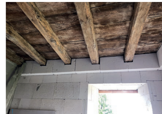
Fig. 6: Upper floor wooden beams
