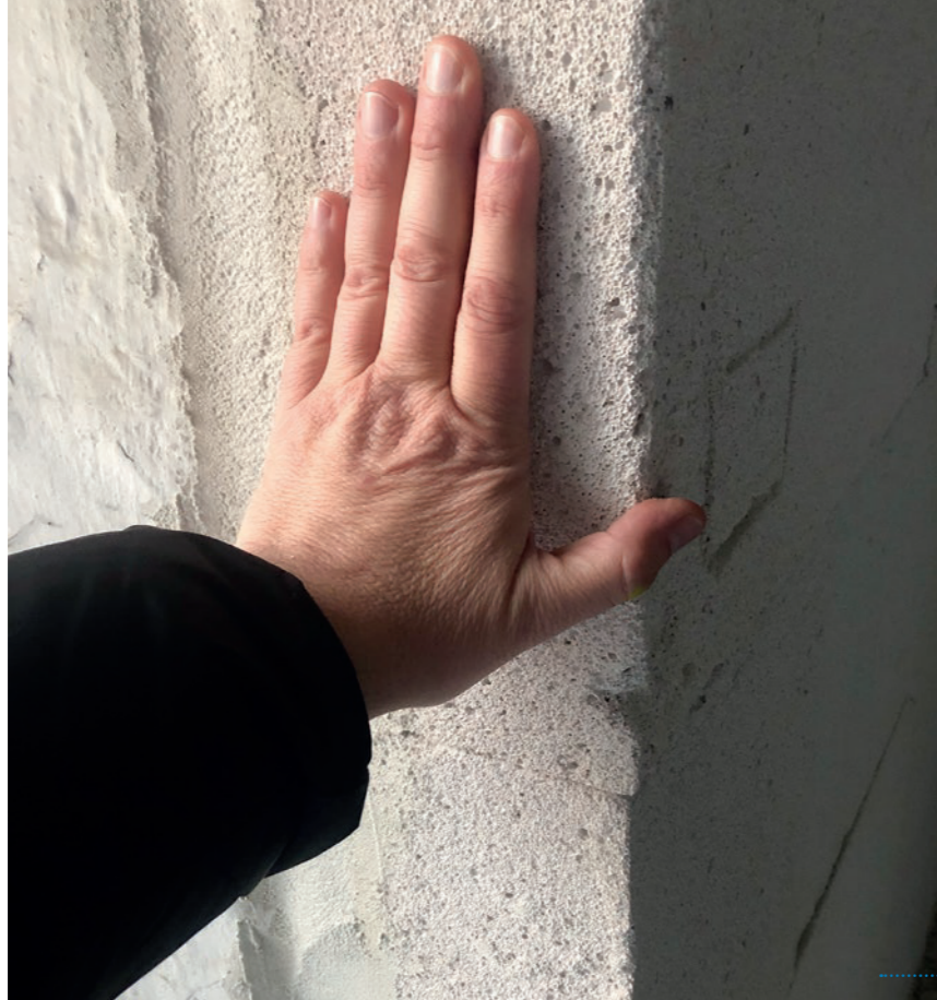
Fig. 3: MultiPOR panels thickness of 140 mm
