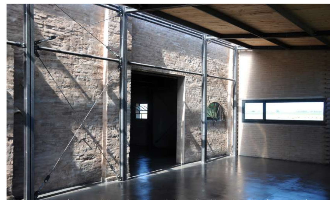
Reconstruction of the completion volume towards the north, with the insertion of new metal frames and floor fabrics smoothed with quartz and treated
