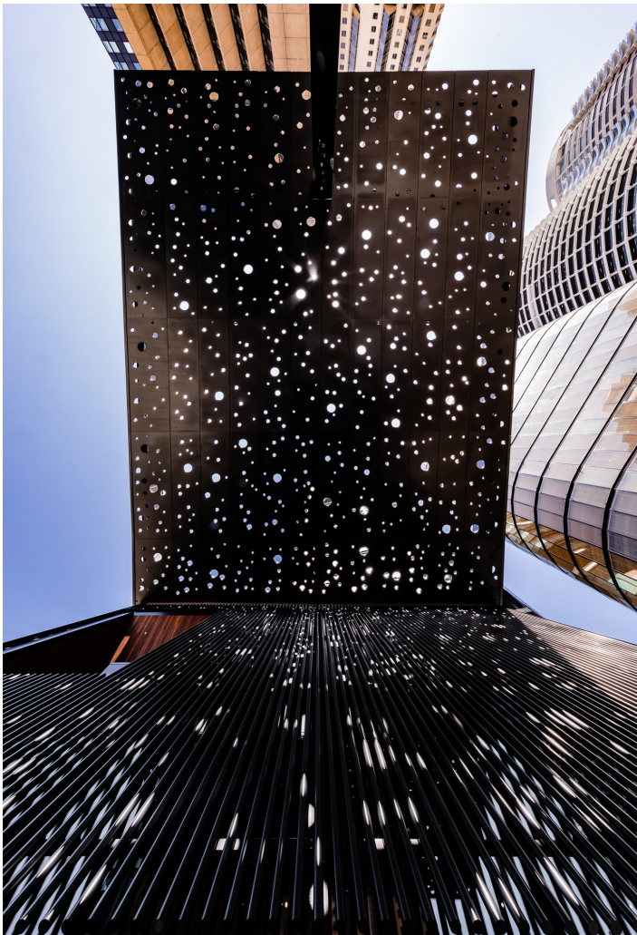
View looking up at perforated canopy which filters dappled light onto the plaza and the facade of the community building
