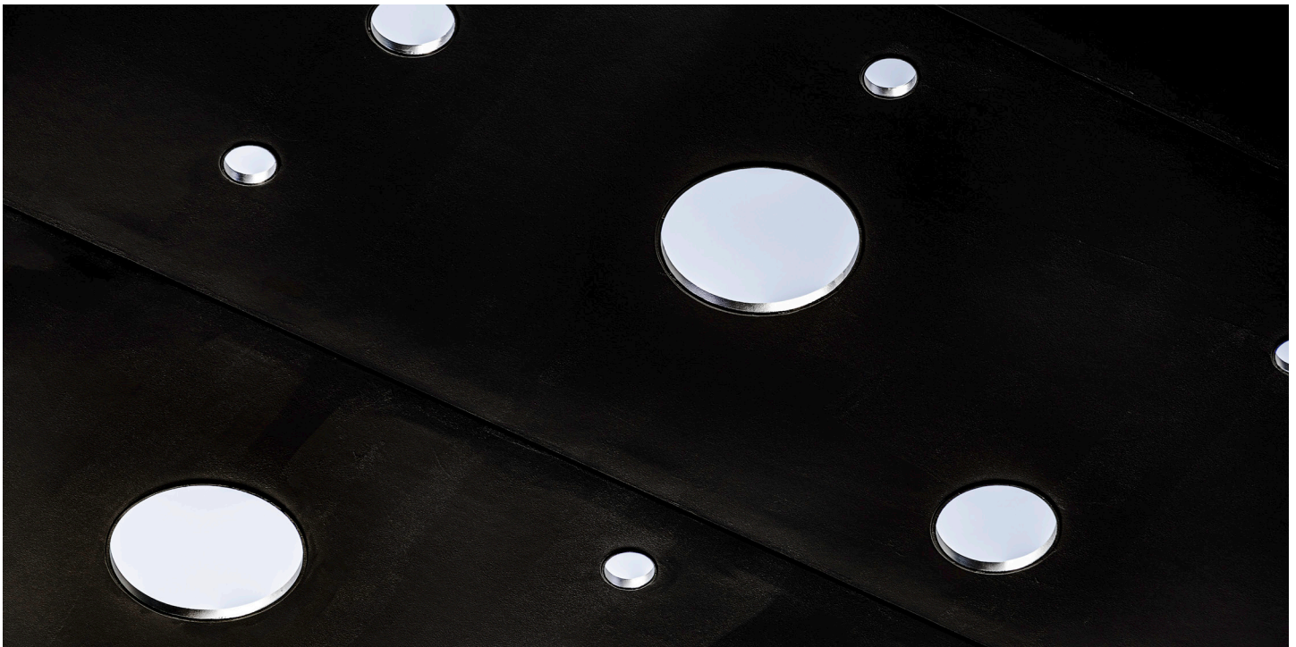
The steel canopy is punctured by mirror-lined openings with views to the sky
